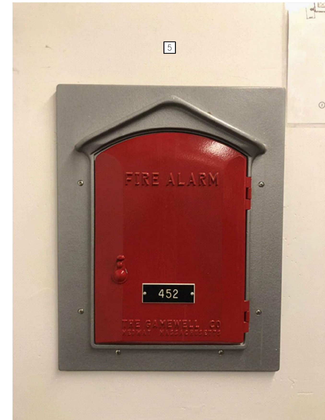
2 CBLS - EXISTING MASTERBOX FIRE ALARM REPORTING SYSTEM ELEVATION IMAGE SCALE: N.T.S.
