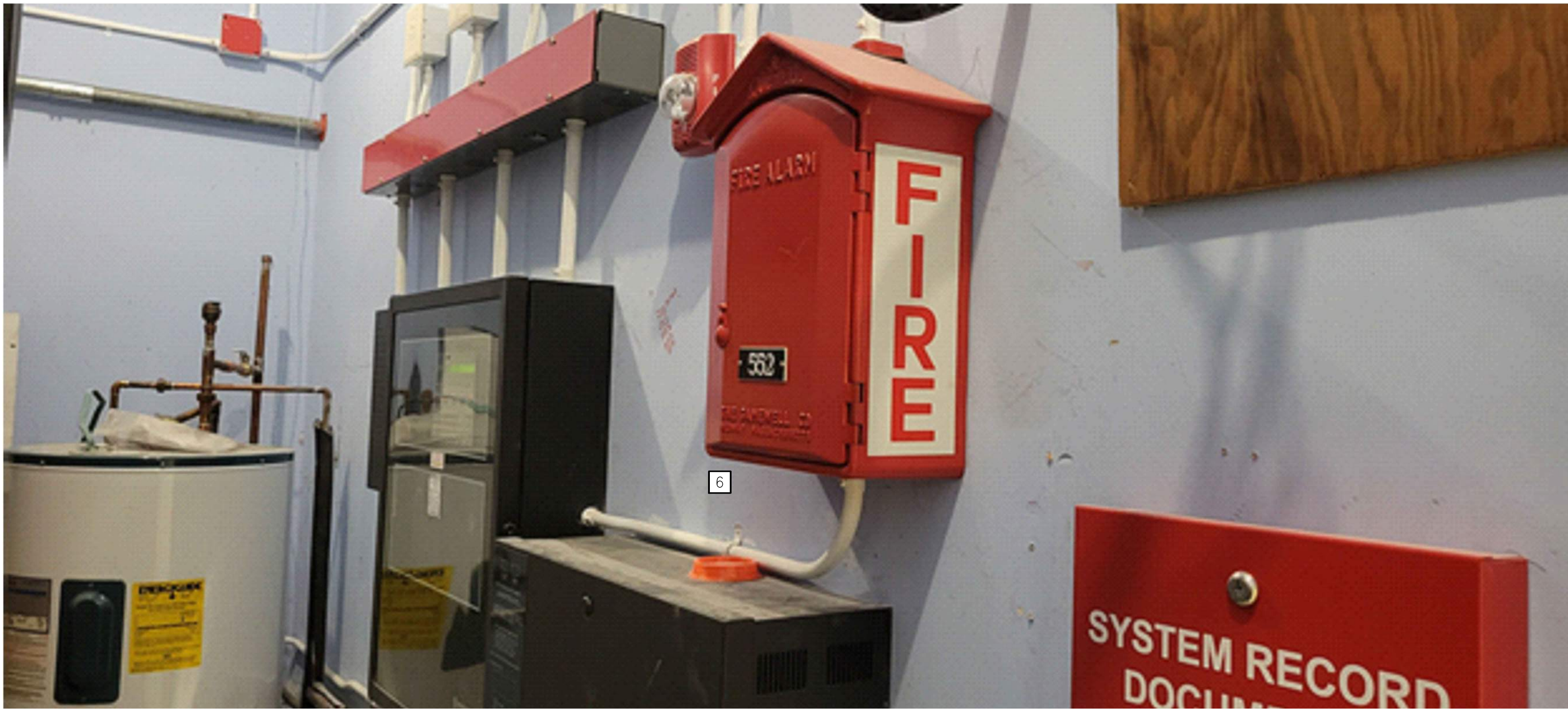
1 GRAD VILLAGE #2 - EXISTING FACP & MASTERBOX FIRE ALARM REPORTING SYSTEM ELEVATION IMAGE SCALE: N.T.S.
