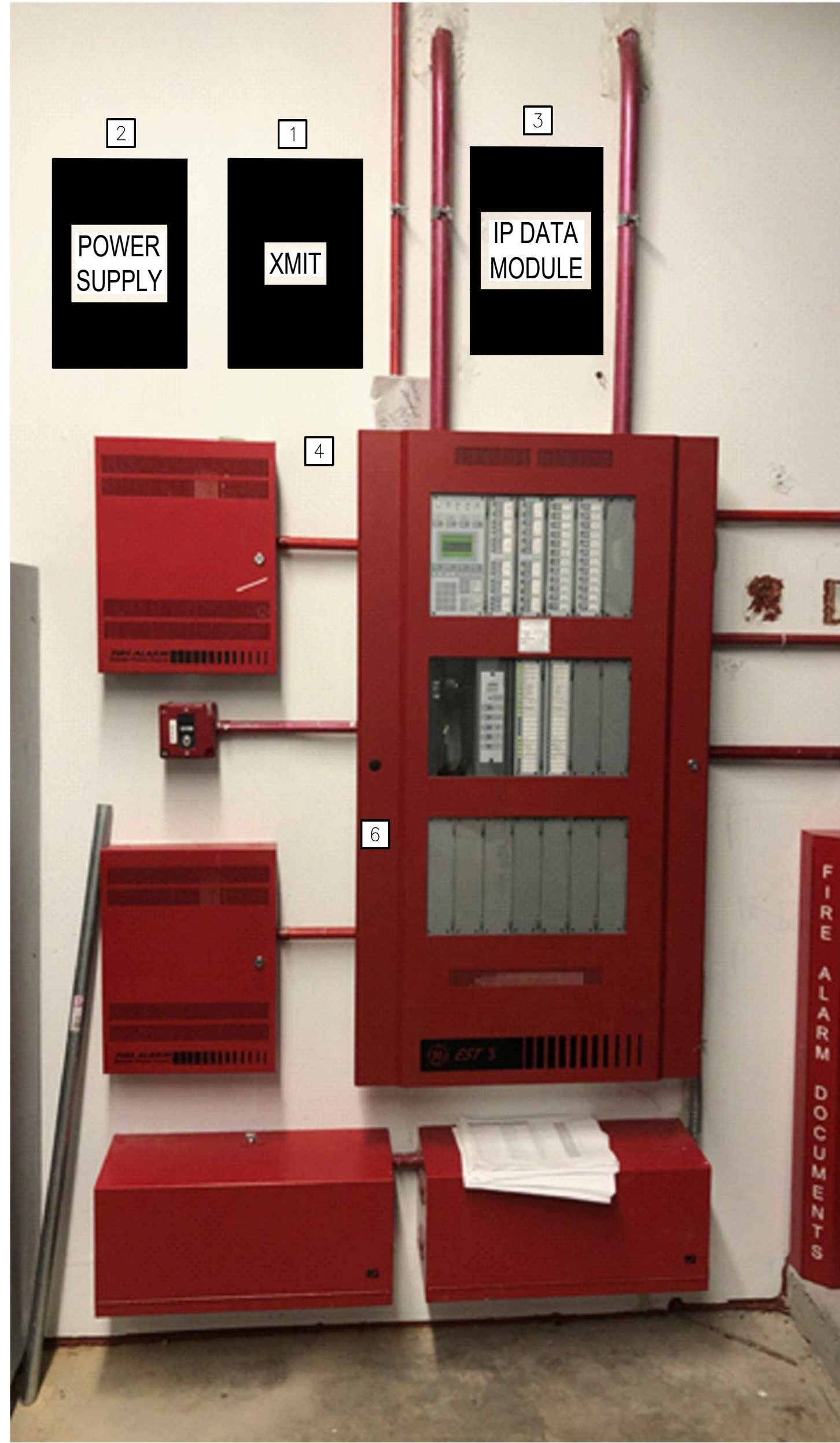
1 CBLS - EXISTING FIRE ALARM CONTROL PANEL FIRE ALARM REPORTING SYSTEM ELEVATION IMAGE SCALE: N.T.S.
