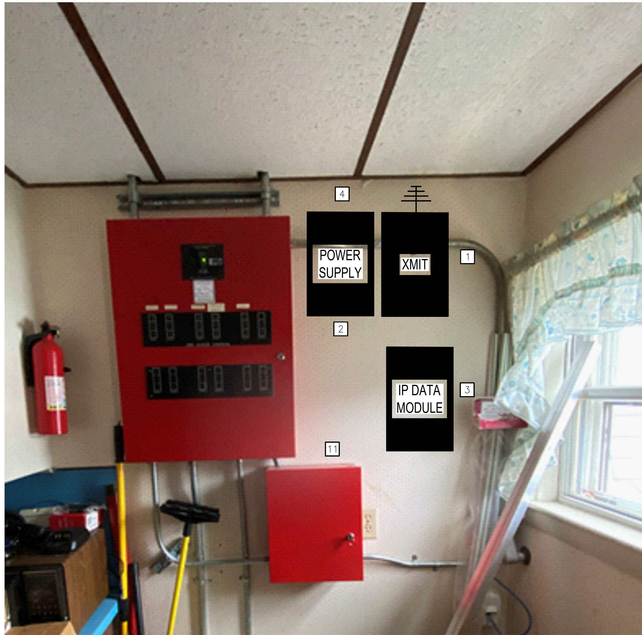
1 FLS - EXISTING FIRE ALARM CONTROL PANEL FIRE ALARM REPORTING SYSTEM ELEVATION IMAGE SCALE: N.T.S.
