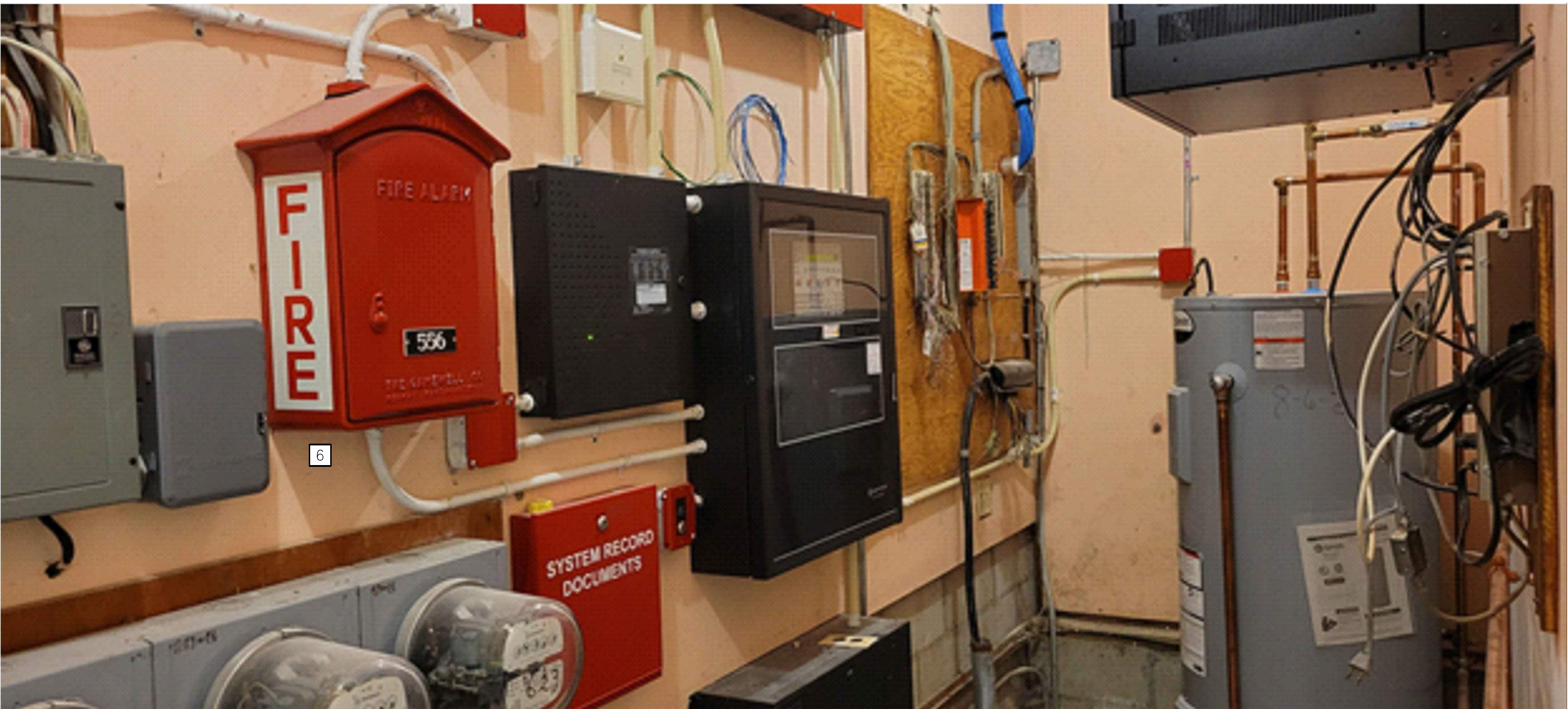
1 GRAD VILLAGE #6 - EXISTING FACP & MASTERBOX FIRE ALARM REPORTING SYSTEM ELEVATION IMAGE SCALE: N.T.S.
