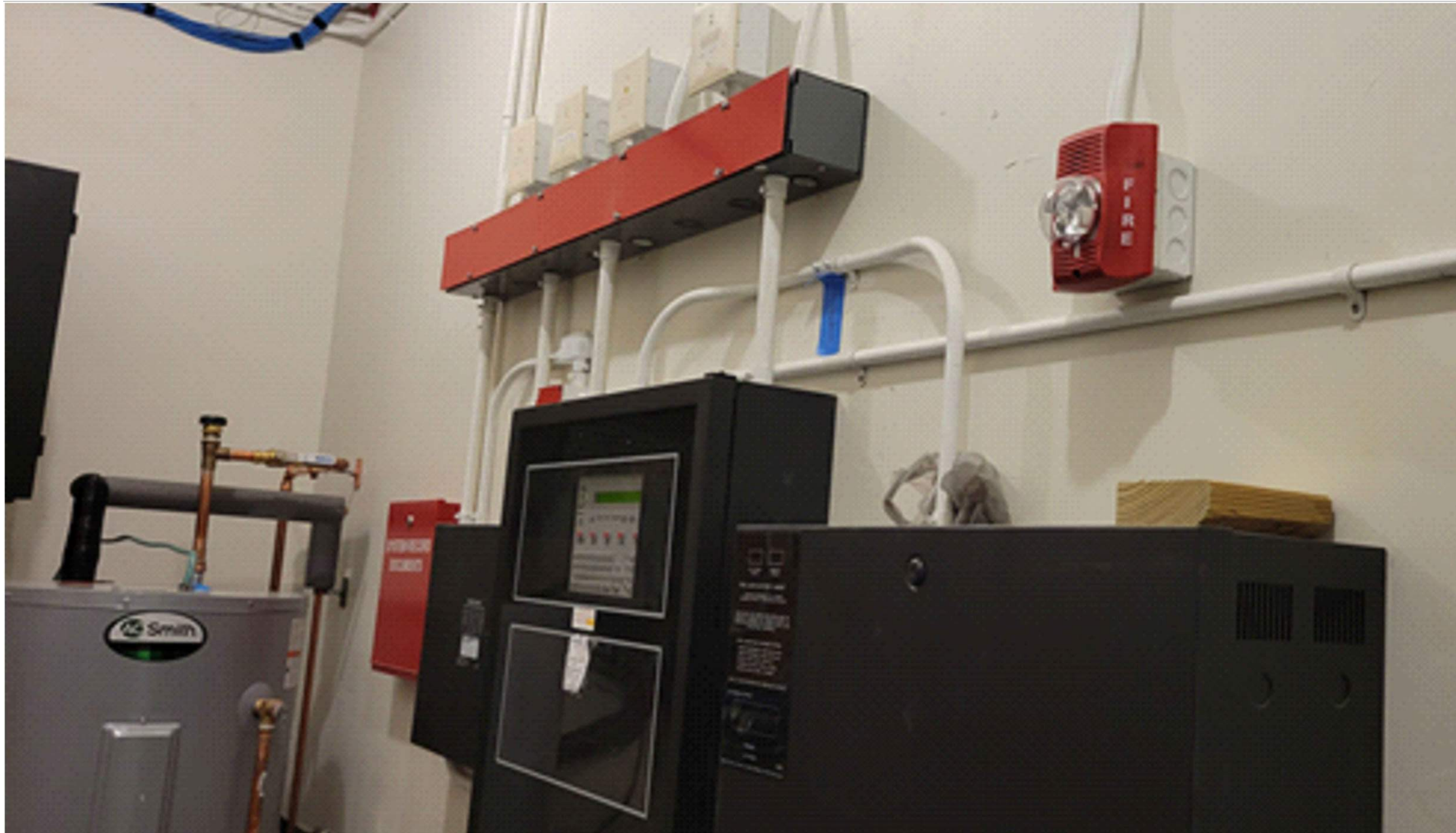
1 GRAD VILLAGE #4 - EXISTING FIRE ALARM CONTROL PANEL FIRE ALARM REPORTING SYSTEM ELEVATION IMAGE SCALE: N.T.S.
