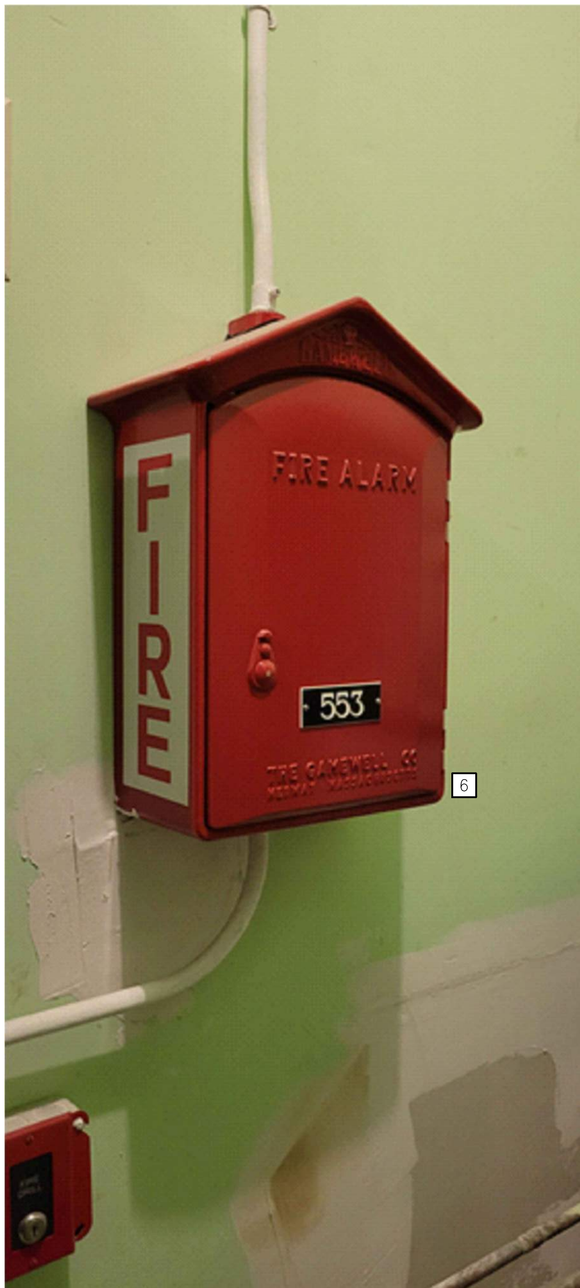
GRAD VILLAGE #3 - EXISTING MASTERBOX FIRE ALARM REPORTING SYSTEM ELEVATION IMAGE SCALE: N.T.S.
