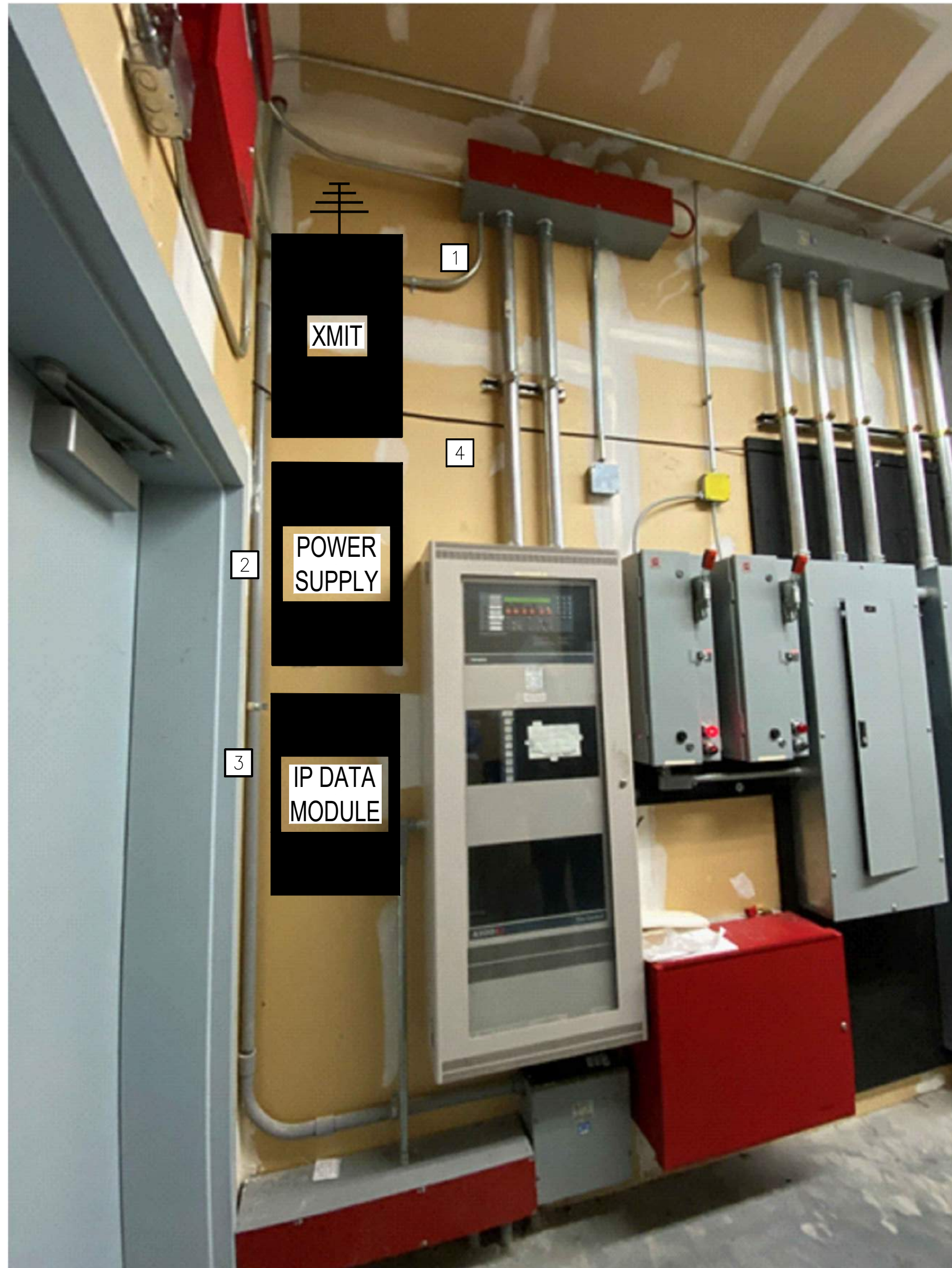
1 BOSS ICE ARENA - EXISTING FIRE ALARM CONTROL PANEL FIRE ALARM REPORTING SYSTEM ELEVATION IMAGE
