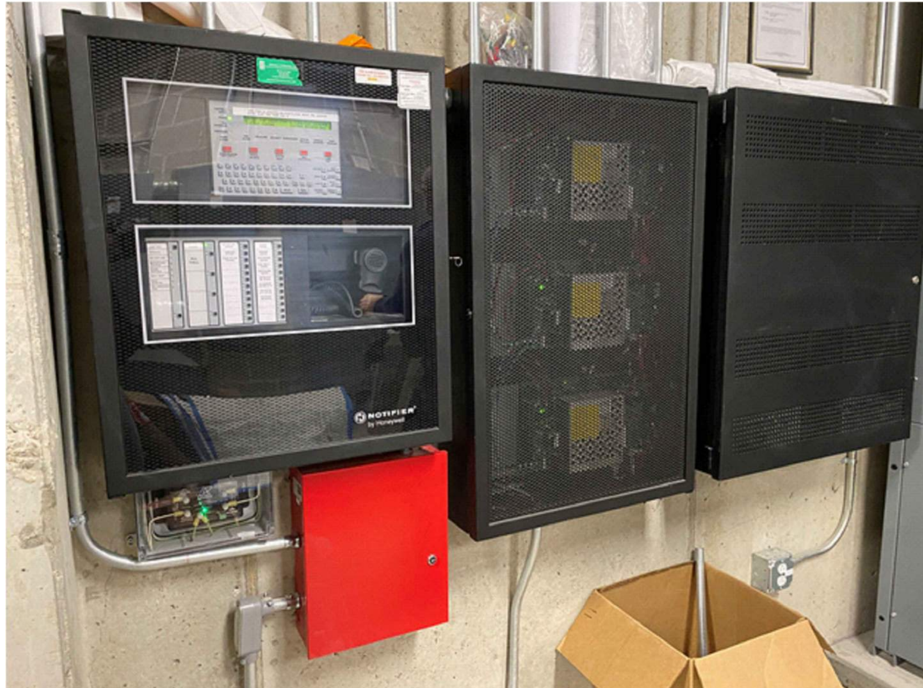
1 BEAUPRE CENTER - EXISTING FIRE ALARM CONTROL PANEL FIRE ALARM REPORTING SYSTEM ELEVATION IMAGE SCALE: N.T.S.
