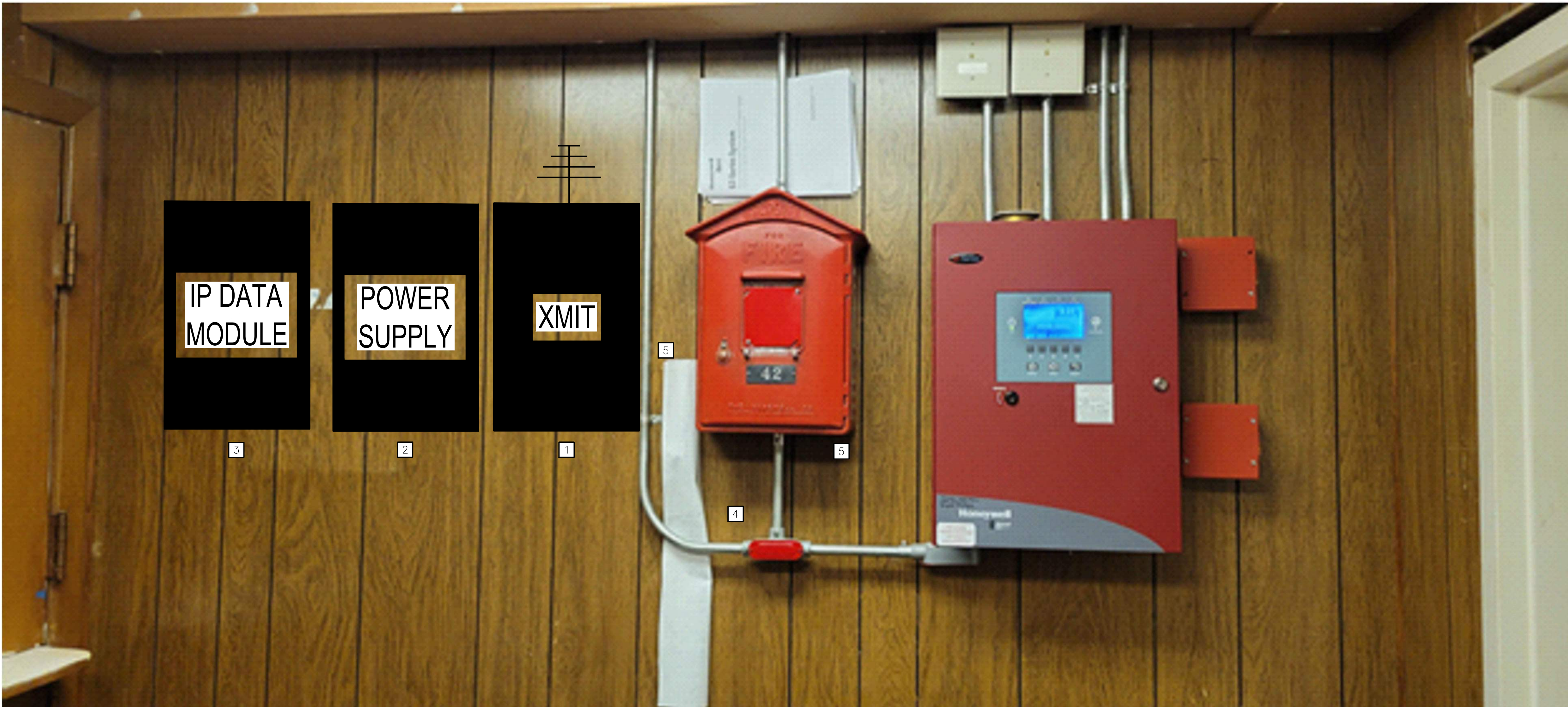
1 UNIVERSITY CLUB - EXISTING FACP & MASTERBOX FIRE ALARM REPORTING SYSTEM ELEVATION IMAGE SCALE: N.T.S.
