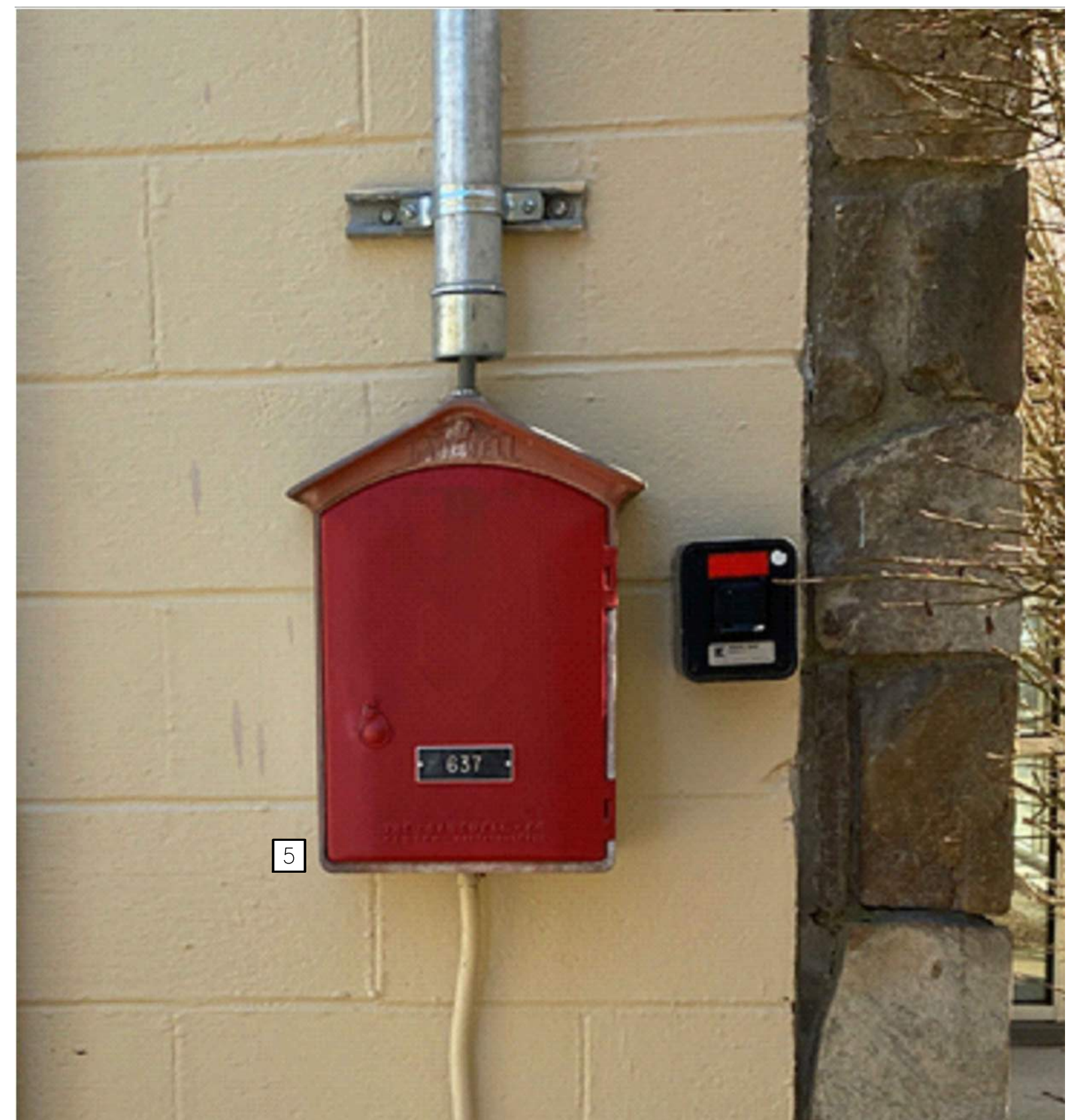
2 POLICE STATION - EXISTING MASTERBOX FIRE ALARM REPORTING SYSTEM ELEVATION IMAGE SCALE: N.T.S.
