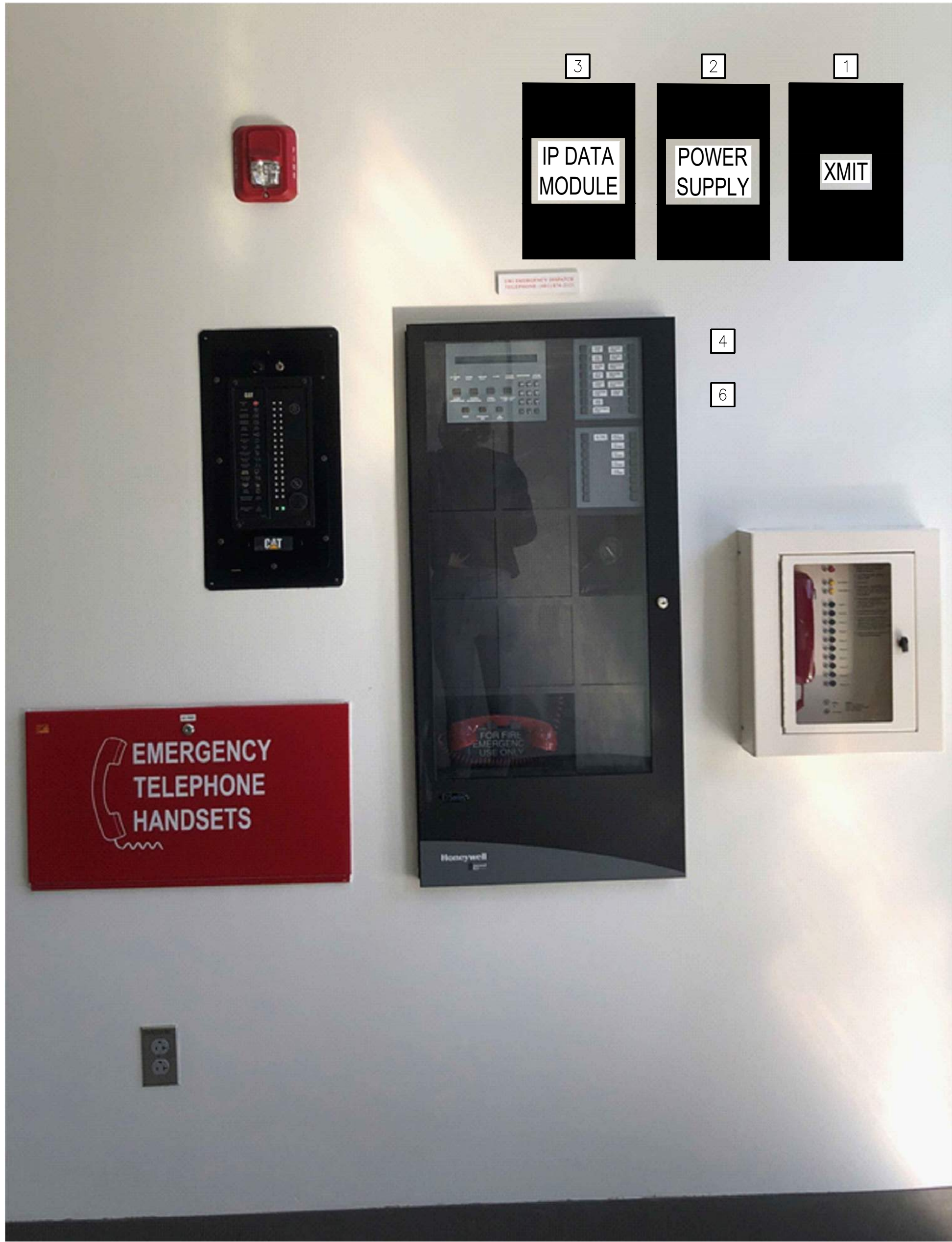
ENGINEERING BUILDING - EXISTING FIRE ALARM CONTROL PANEL FIRE ALARM REPORTING SYSTEM ELEVATION IMAGE
