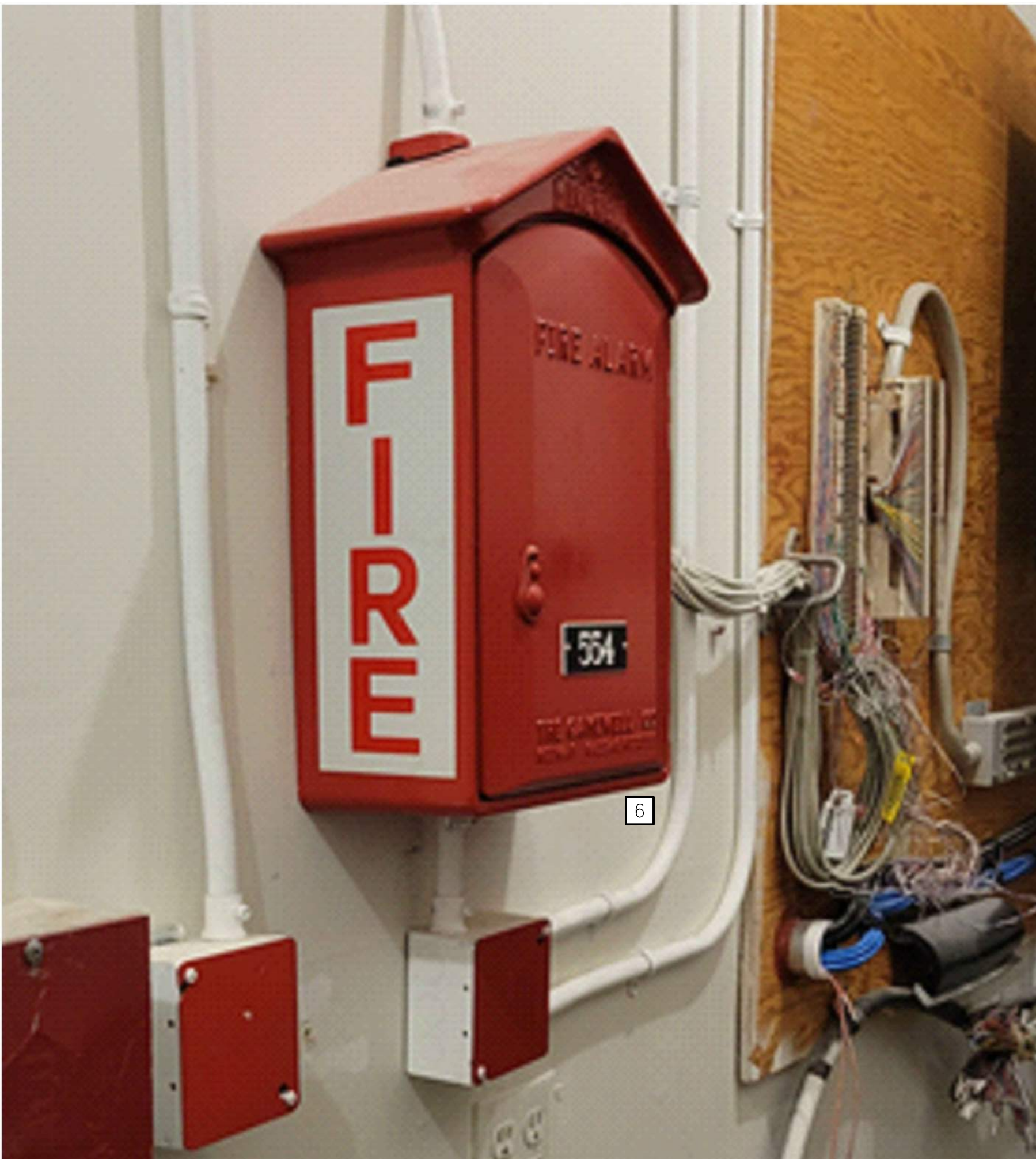
2 GRAD VILLAGE #4 - EXISTING MASTERBOX FIRE ALARM REPORTING SYSTEM ELEVATION IMAGE SCALE: N.T.S.
