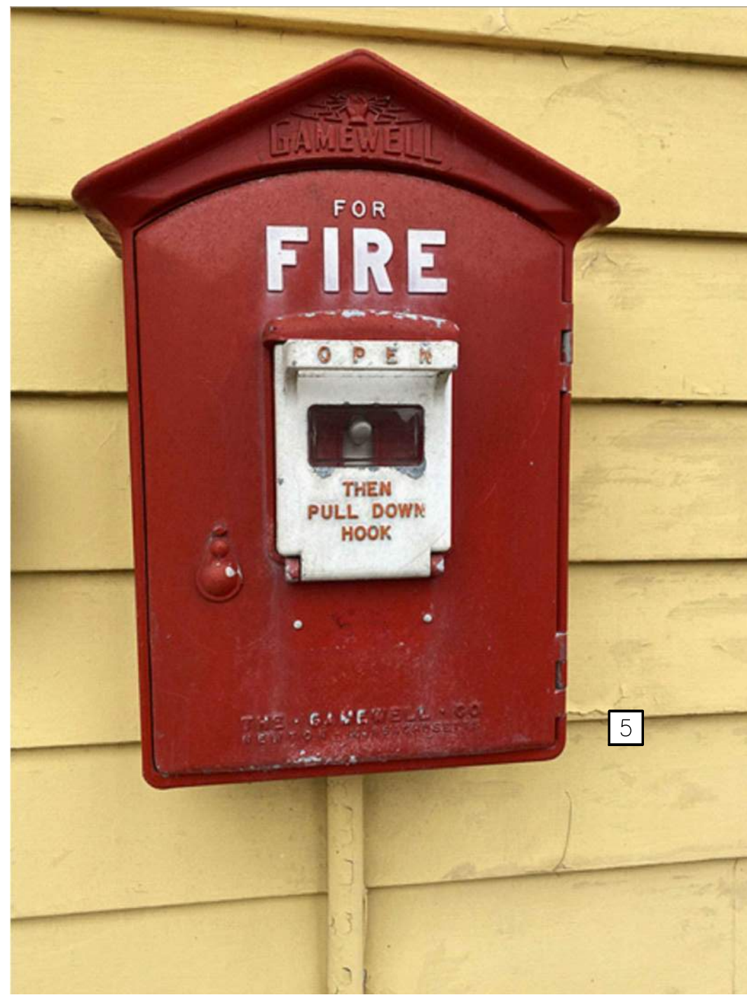
2 WOMEN'S CENTER - EXISTING MASTERBOX FIRE ALARM REPORTING SYSTEM ELEVATION IMAGE SCALE: N.T.S.
