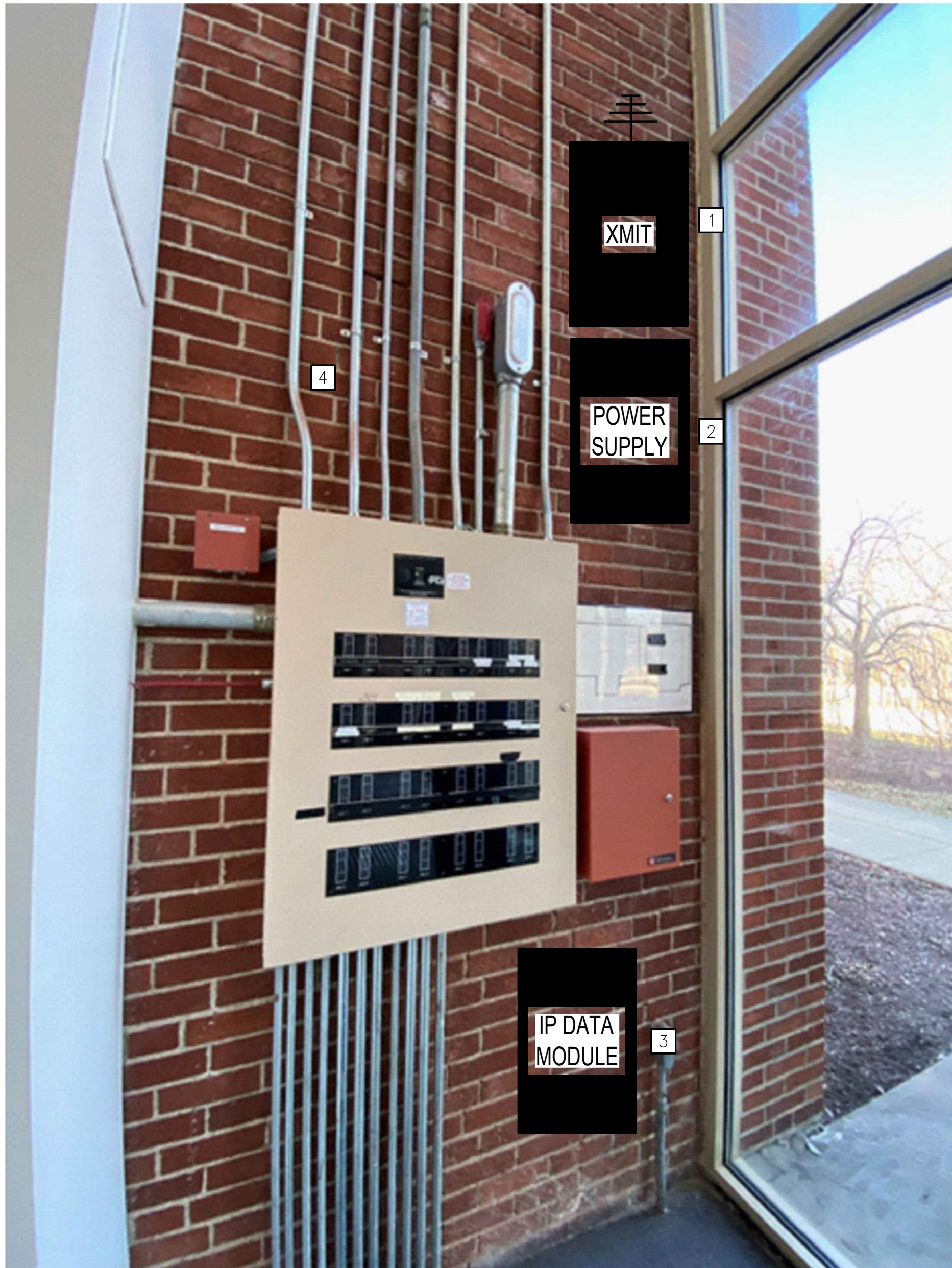
1 MACKAL FIELDHOUSE - EXISTING FIRE ALARM CONTROL PANEL FIRE ALARM REPORTING SYSTEM ELEVATION IMAGE SCALE: N.T.S.
