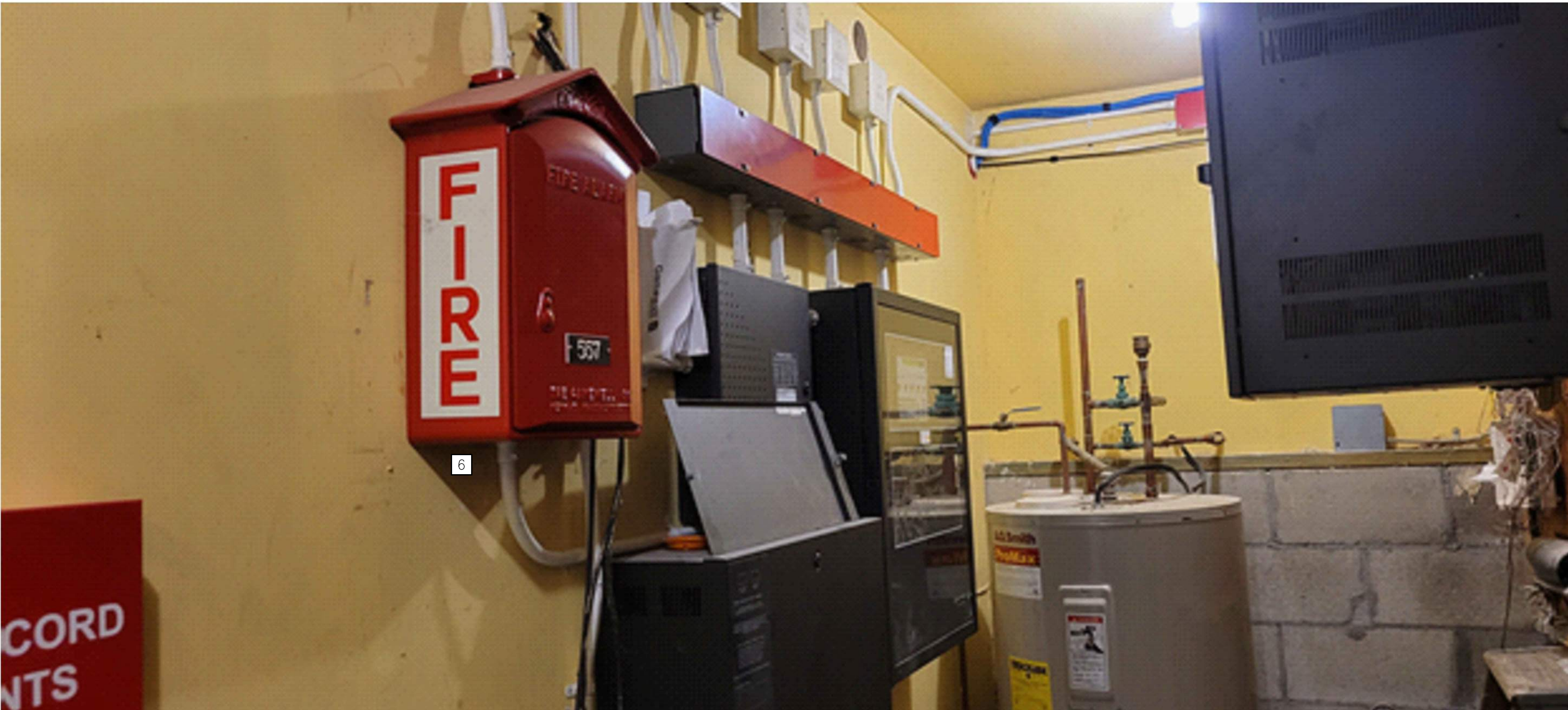
1 GRAD VILLAGE #7 - EXISTING FIRE ALARM CONTROL PANEL FIRE ALARM REPORTING SYSTEM ELEVATION IMAGE SCALE: N.T.S.
