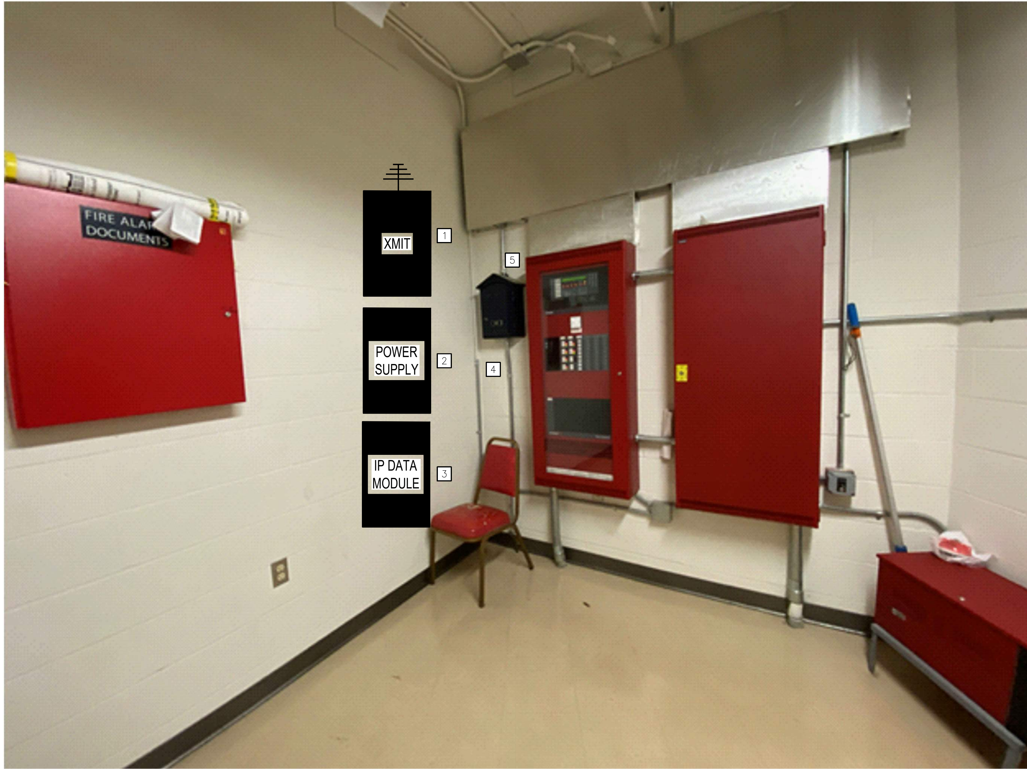
1 WILEY HALL - EXISTING FACP & MASTERBOX FIRE ALARM REPORTING SYSTEM ELEVATION IMAGE SCALE: N.T.S.
