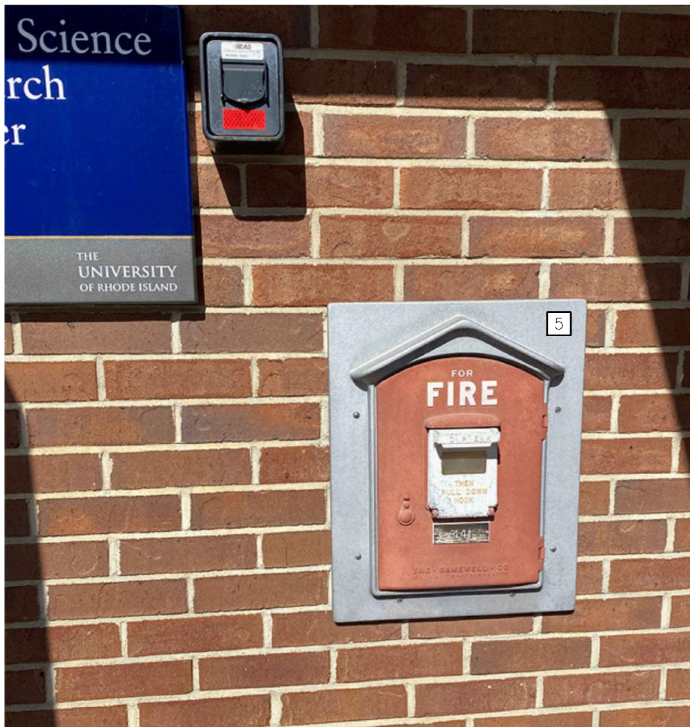
2 SSRC - EXISTING MASTERBOX FIRE ALARM REPORTING SYSTEM ELEVATION IMAGE SCALE: N.T.S.
