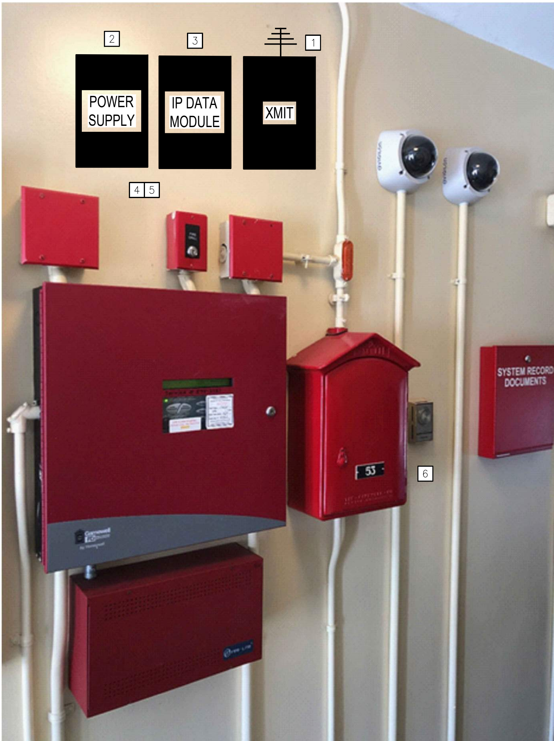
GATEWAY APT #2 - FIRE ALARM CONTROL PANEL FIRE ALARM REPORTING SYSTEM ELEVATION IMAGE SCALE: N.T.S.
