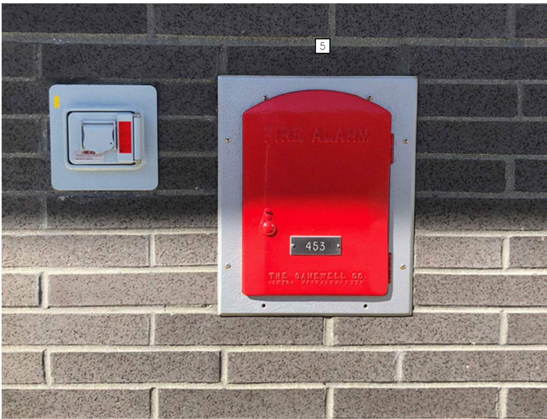
ENGINEERING BUILDING - EXISTING MASTERBOX FIRE ALARM REPORTING SYSTEM ELEVATION IMAGE
