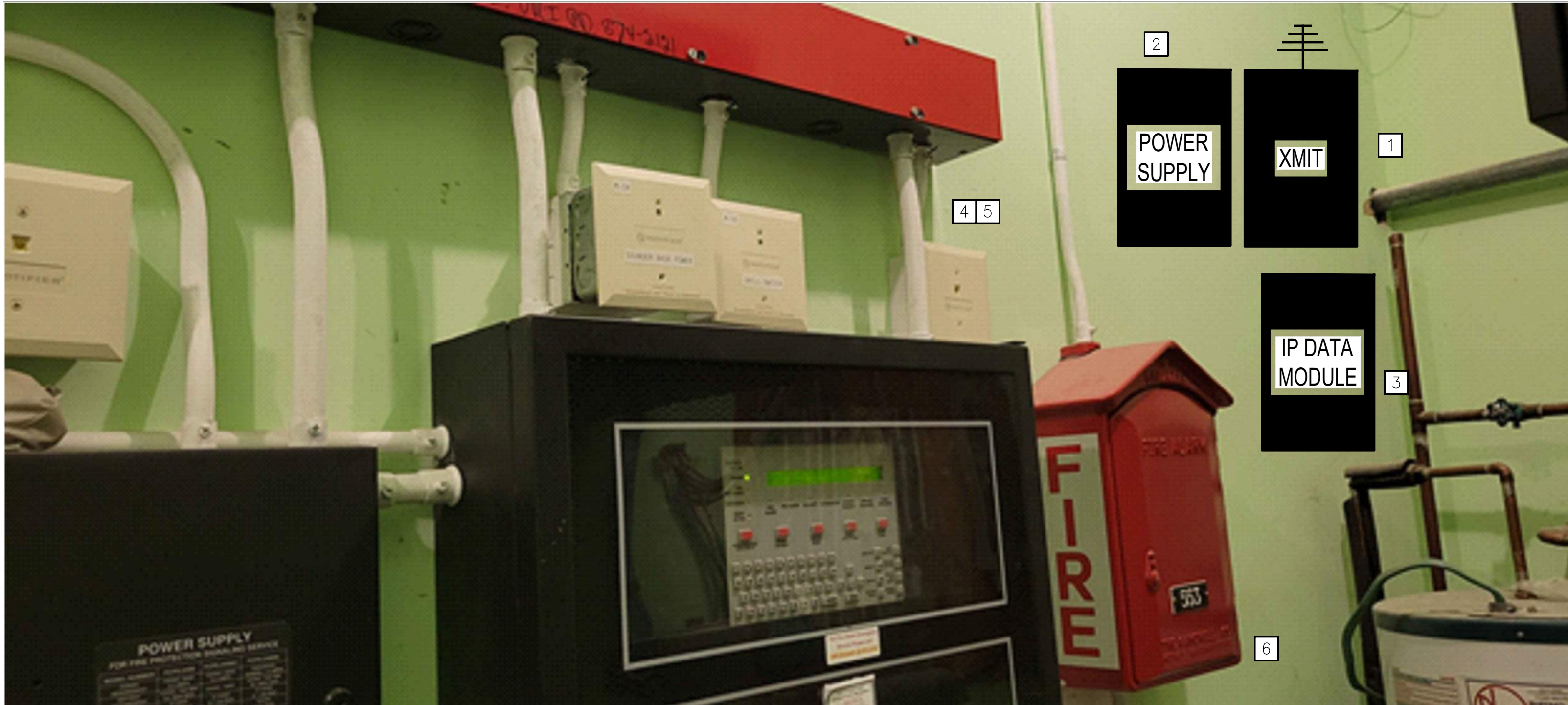
GRAD VILLAGE #3 - EXISTING FIRE ALARM CONTROL PANEL FIRE ALARM REPORTING SYSTEM ELEVATION IMAGE SCALE: N.T.S.
