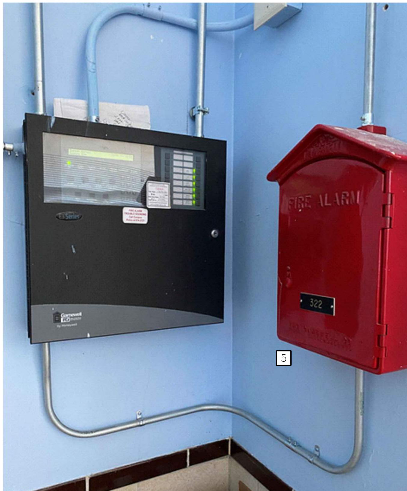
2 KEANEY GYMNASIUM - EXISTING MASTERBOX FIRE ALARM REPORTING SYSTEM ELEVATION IMAGE
