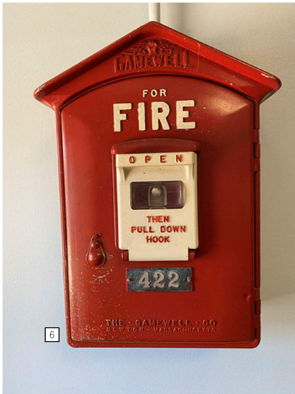
2 KINGSTON FIRE - EXISTING MASTERBOX FIRE ALARM REPORTING SYSTEM ELEVATION IMAGE SCALE: N.T.S.
