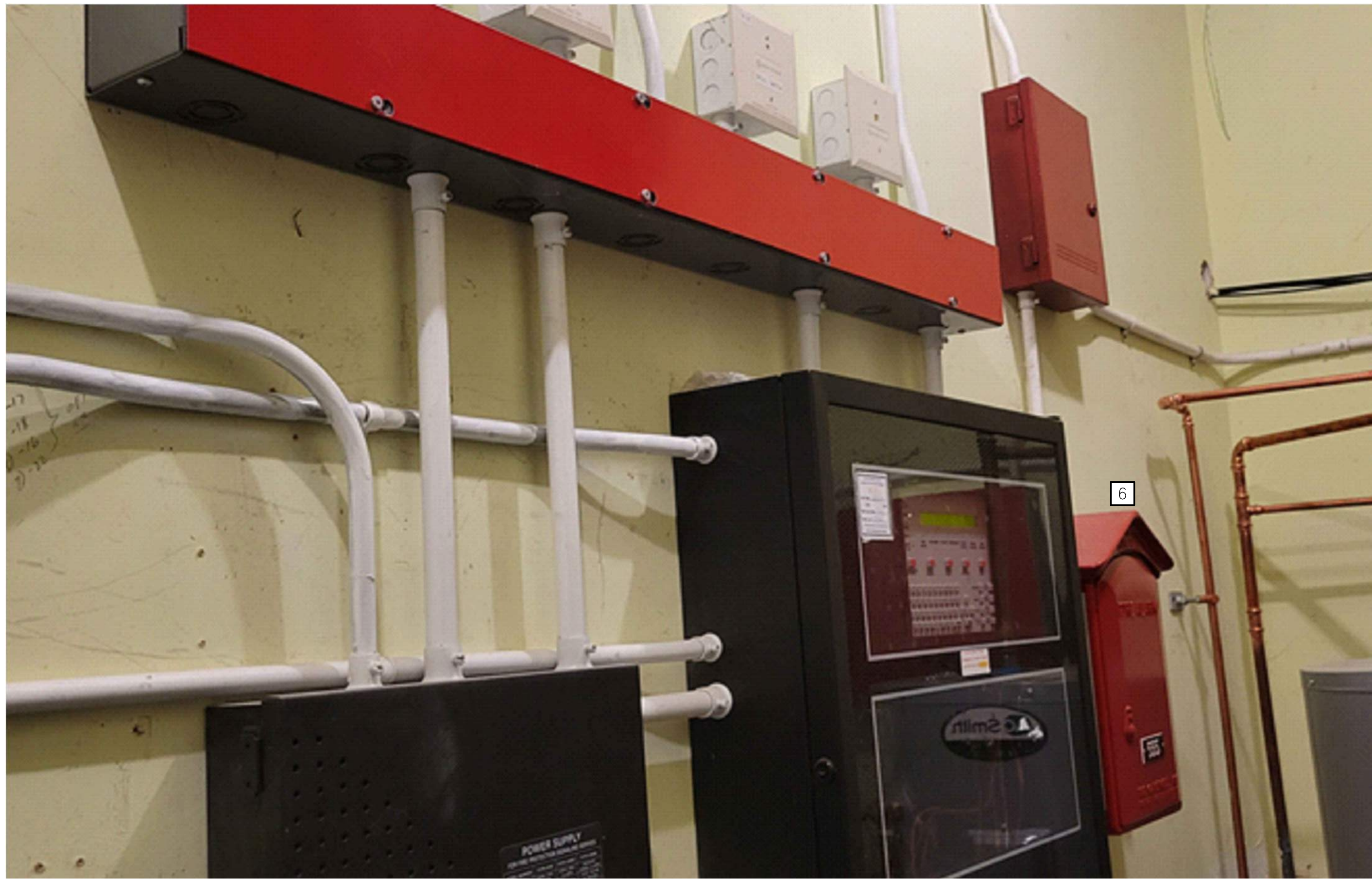
1 GRAD VILLAGE #5 - EXISTING FACP & MASTERBOX FIRE ALARM REPORTING SYSTEM ELEVATION IMAGE SCALE: N.T.S.
