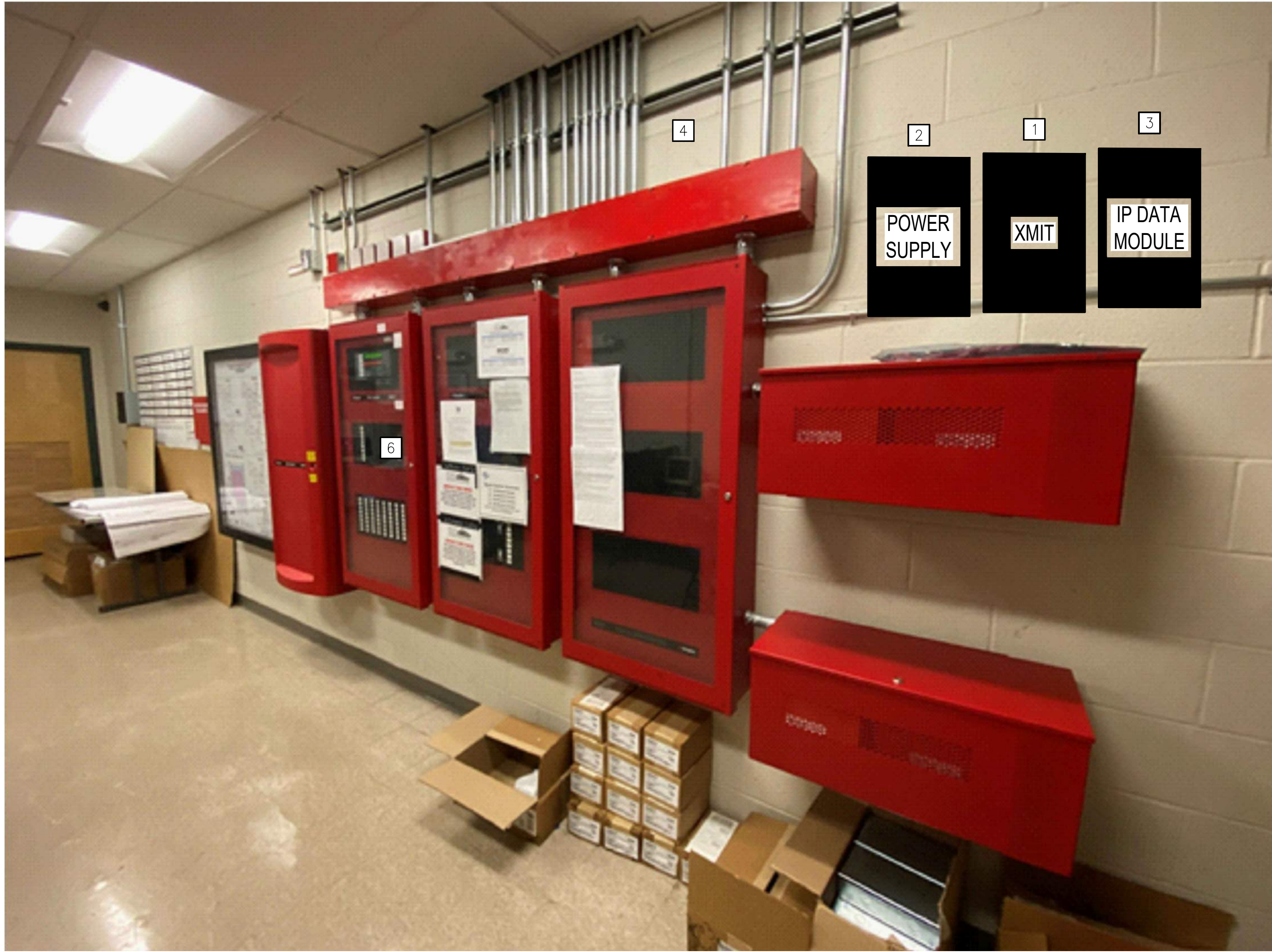
1 RYAN CENTER - EXISTING FIRE ALARM CONTROL PANEL FIRE ALARM REPORTING SYSTEM ELEVATION IMAGE SCALE: N.T.S.
