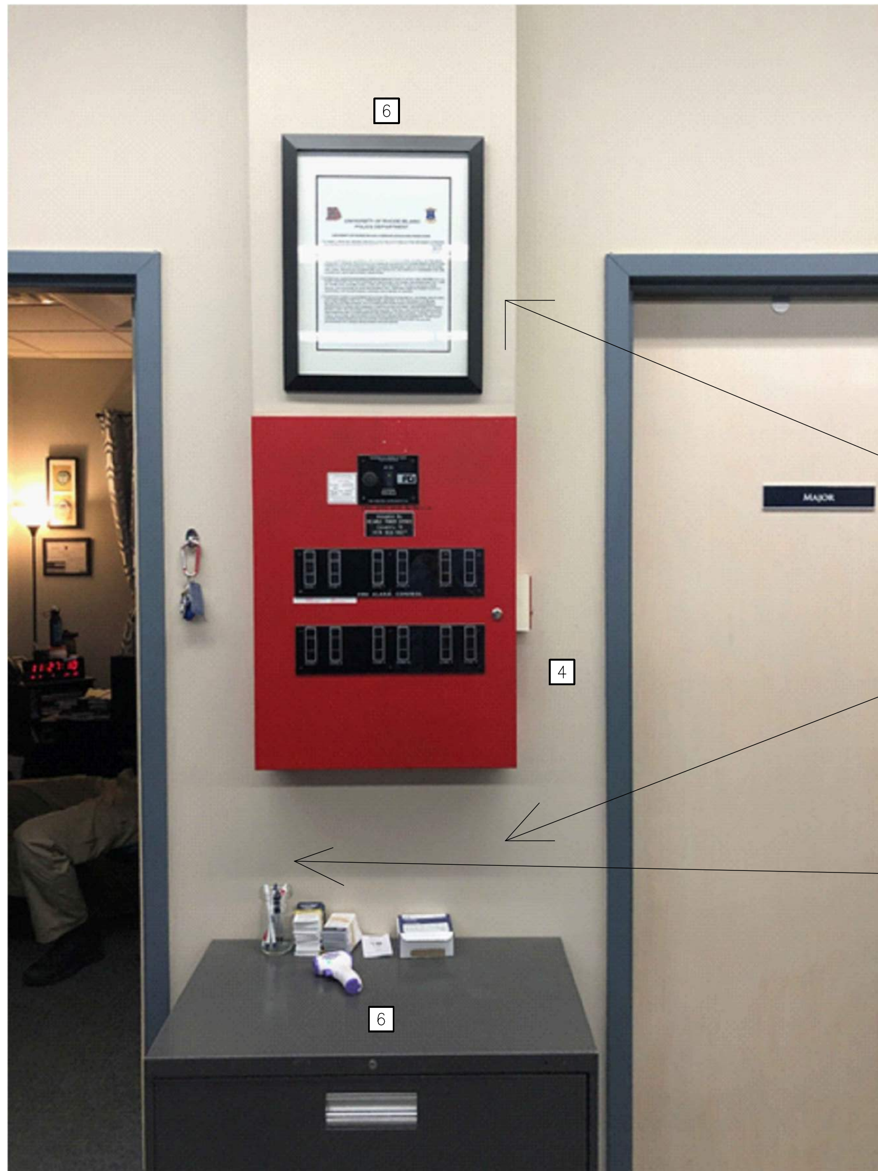
1 POLICE STATION - EXISTING FIRE ALARM CONTROL PANEL FIRE ALARM REPORTING SYSTEM ELEVATION IMAGE SCALE: N.T.S.
