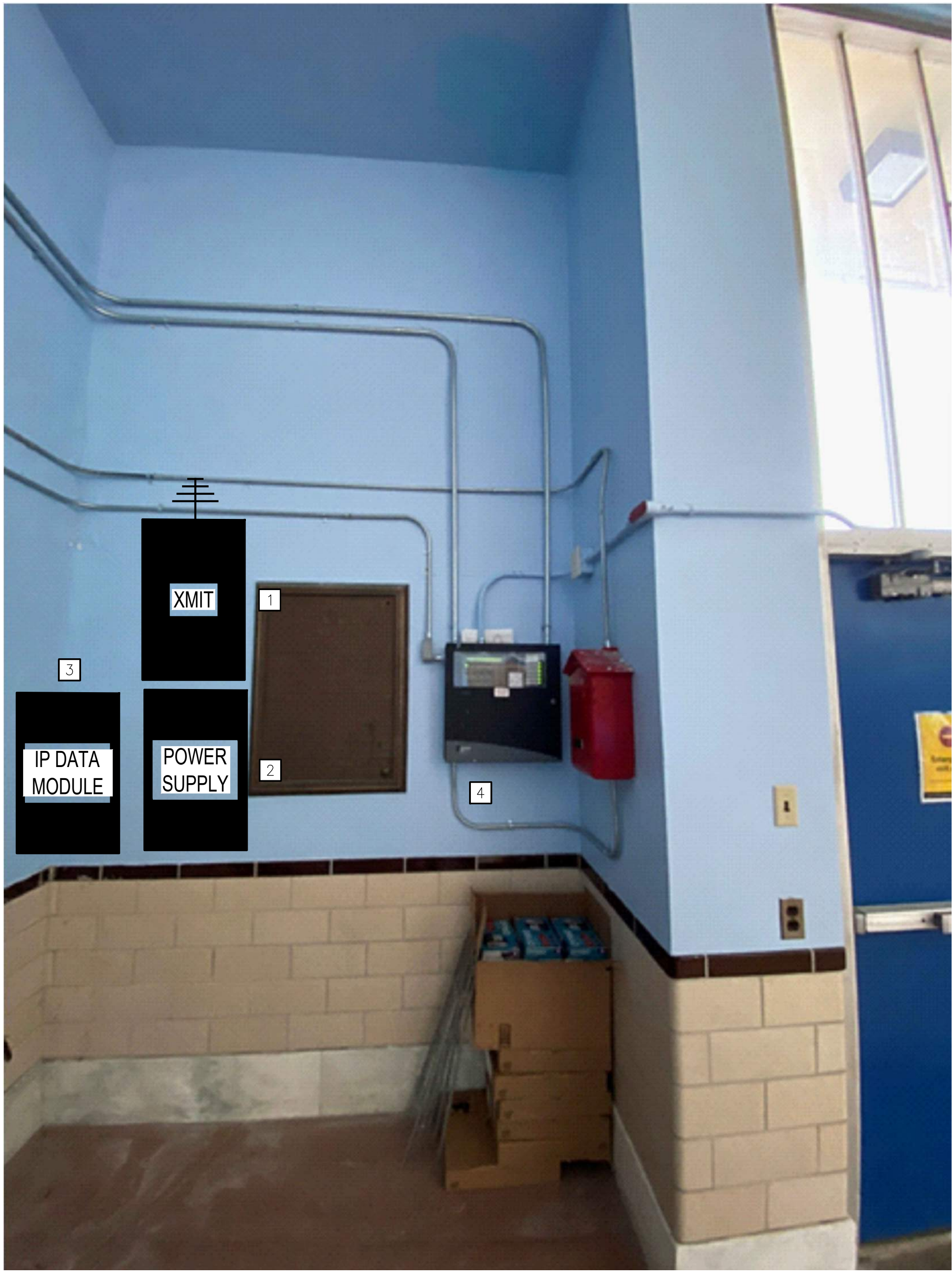
1 KEANEY GYMNASIUM - EXISTING FIRE ALARM CONTROL PANEL FIRE ALARM REPORTING SYSTEM ELEVATION IMAGE
