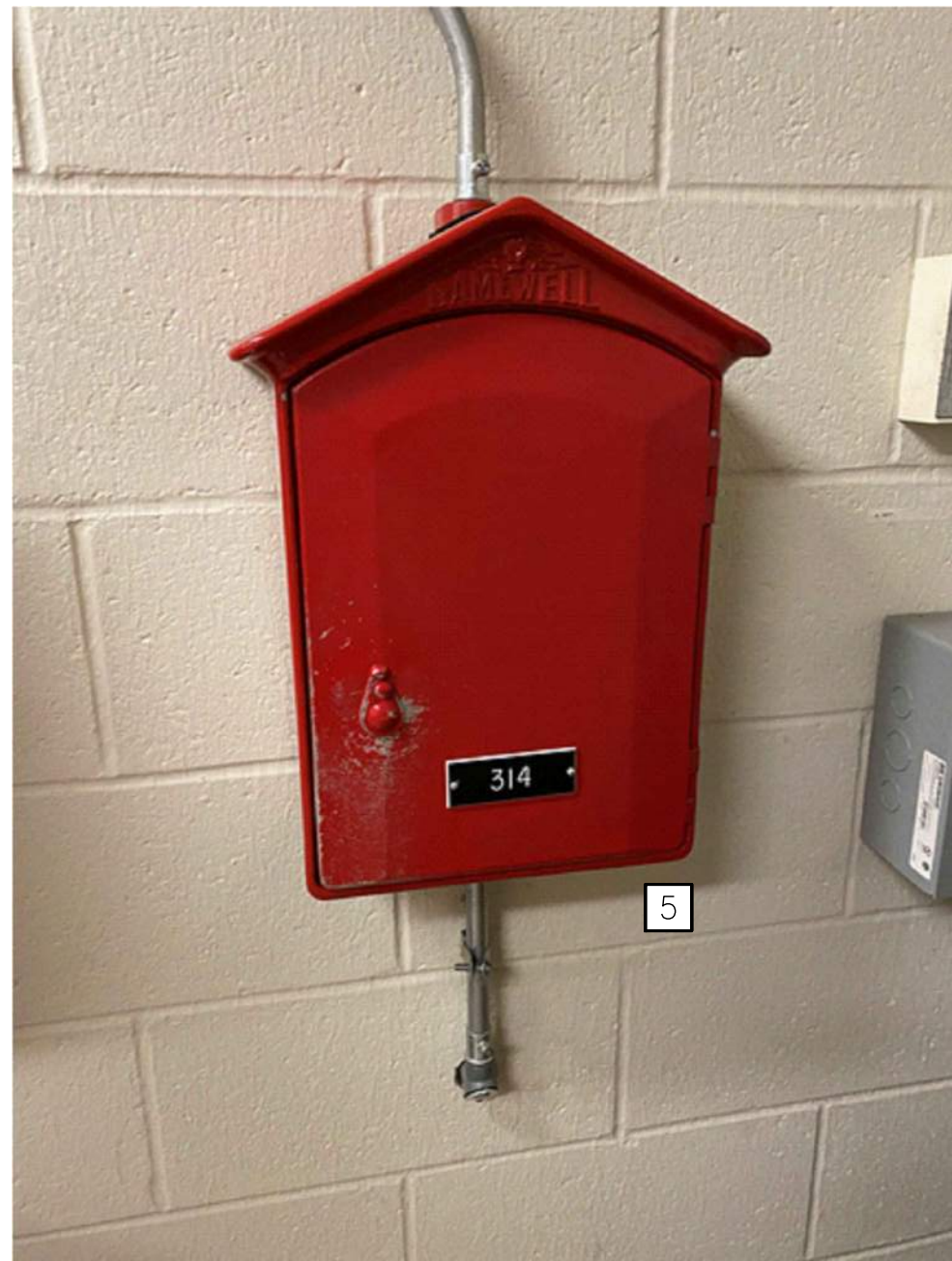
2 RYAN CENTER - EXISTING MASTERBOX FIRE ALARM REPORTING SYSTEM ELEVATION IMAGE SCALE: N.T.S.
