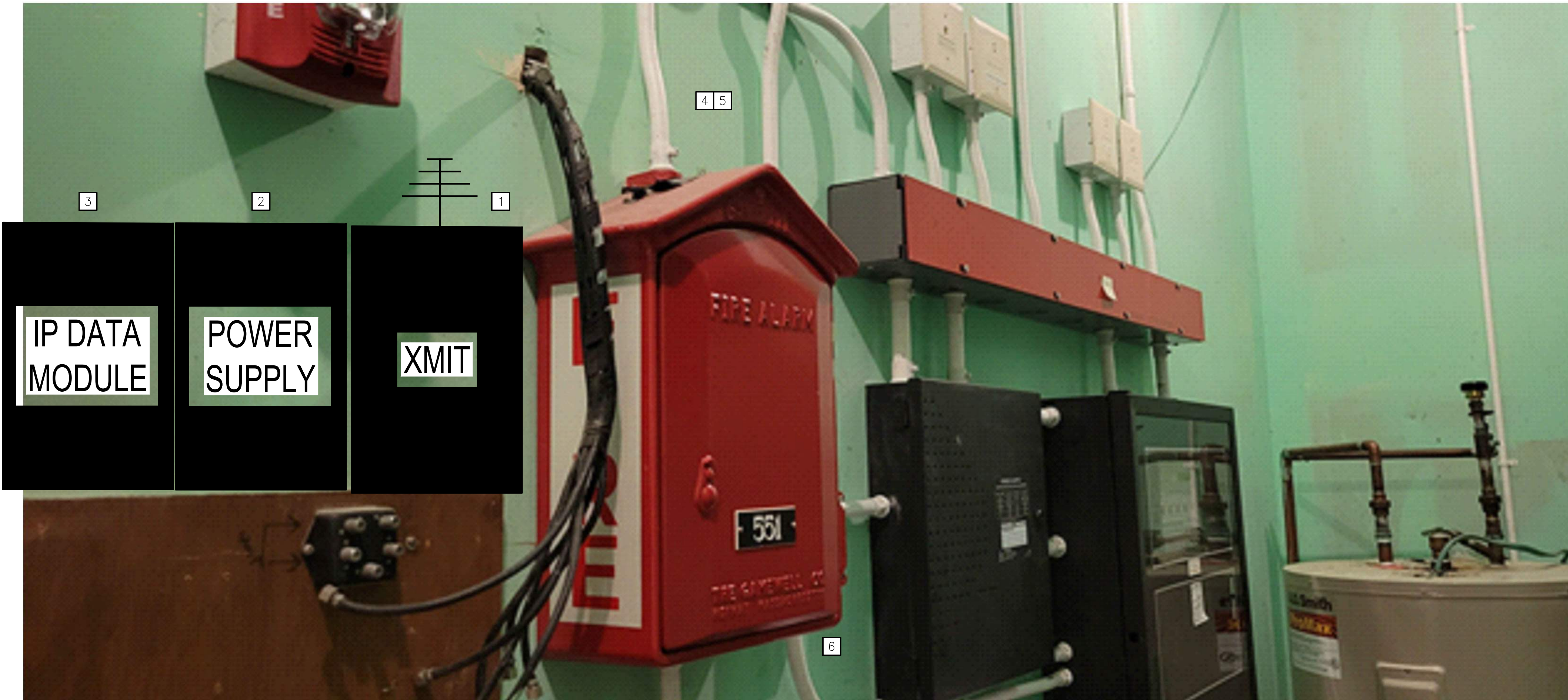
1 GRAD VILLAGE #1 - EXISTING FACP & MASTERBOX FIRE ALARM REPORTING SYSTEM ELEVATION IMAGE SCALE: N.T.S.
