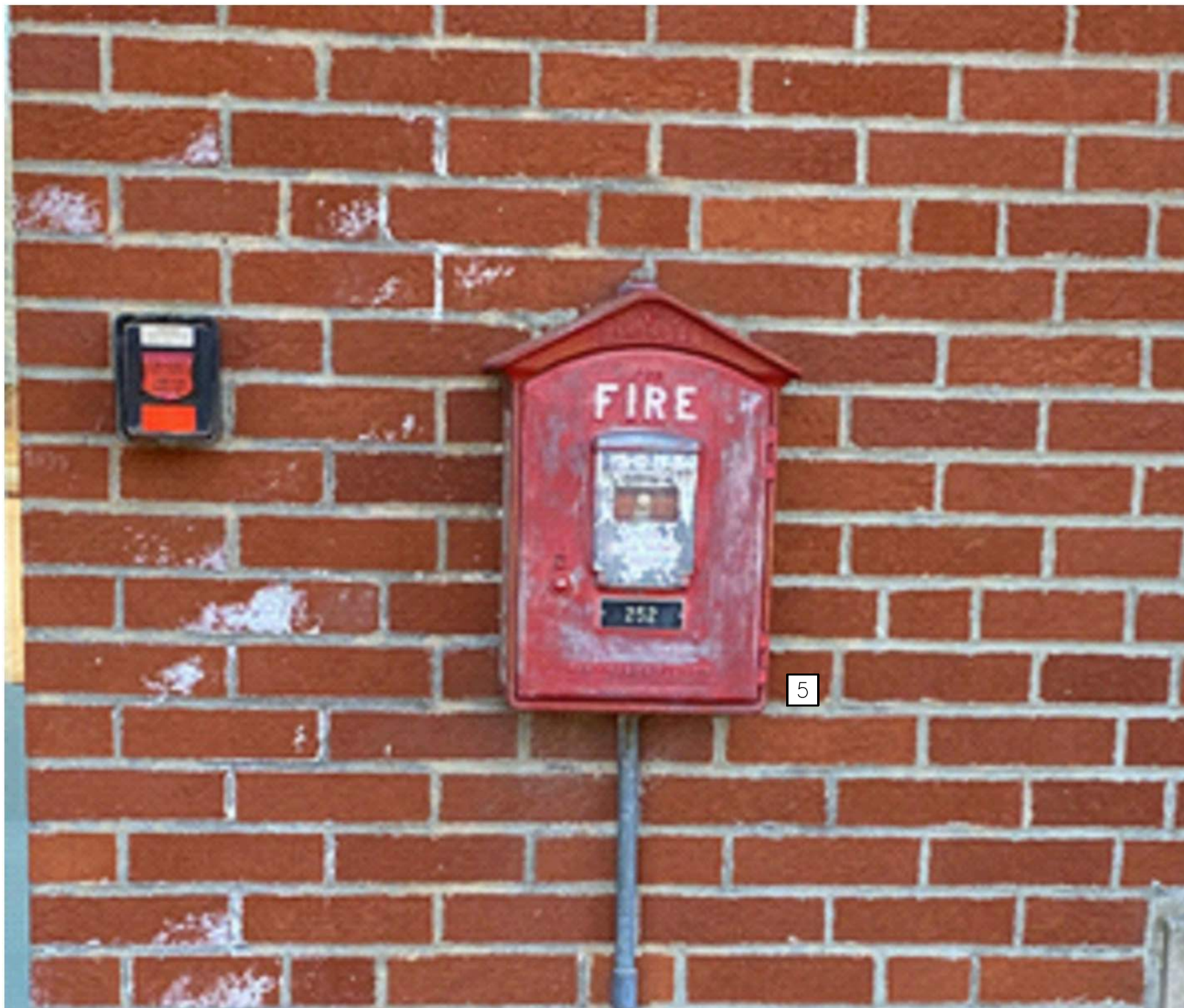
2 MACKAL FIELDHOUSE - EXISTING MASTERBOX FIRE ALARM REPORTING SYSTEM ELEVATION IMAGE SCALE: N.T.S.
